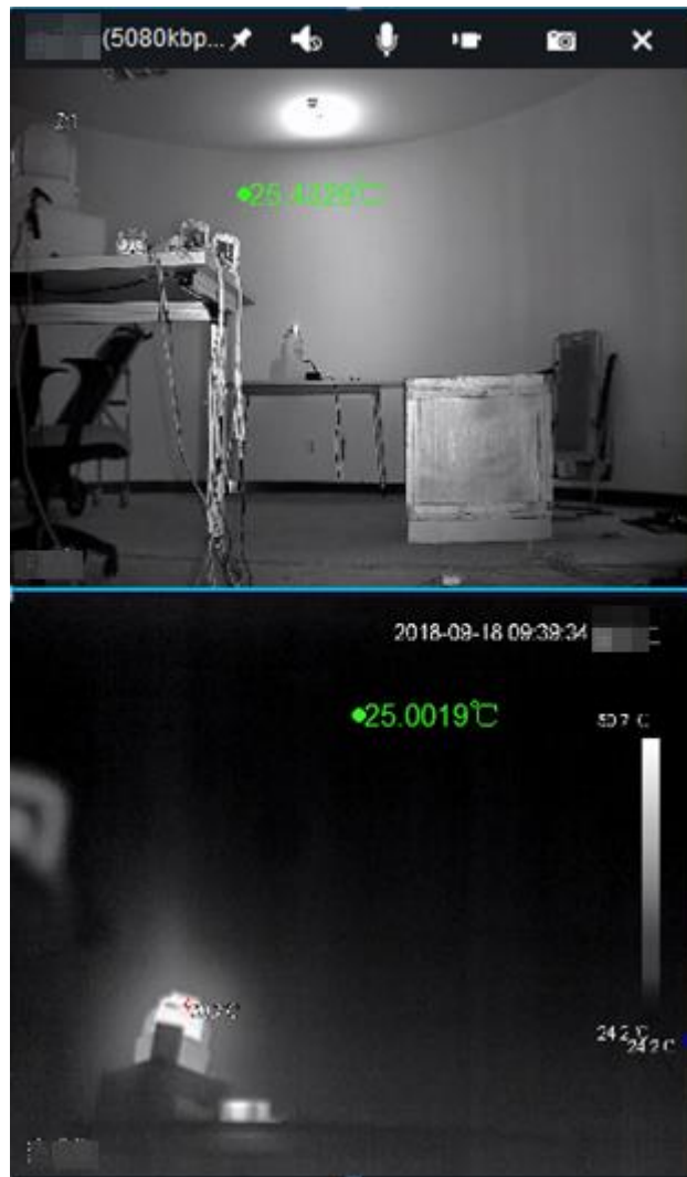
Figure 4-304 Real-time temperature measurement
